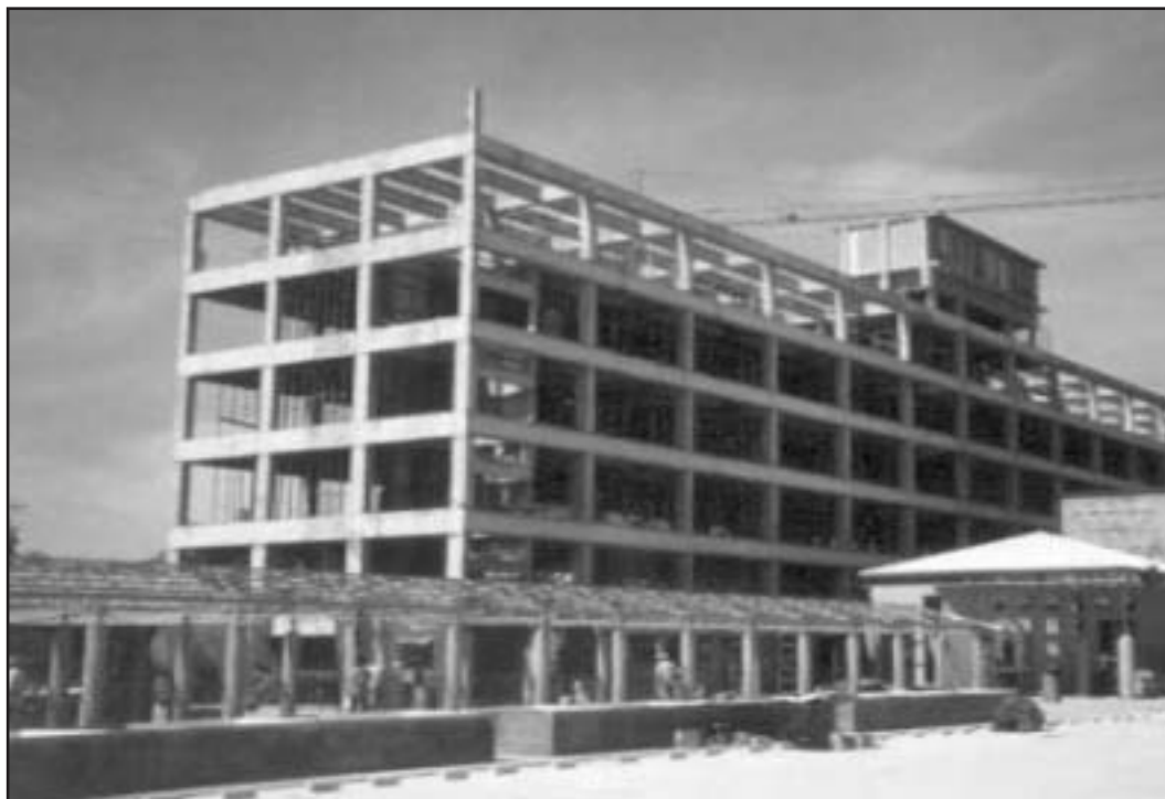
Retrofitted hospital Photo: Osorio, PAHO
