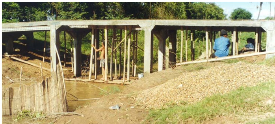
A low cost bridge built through community based action in Cambodia.
